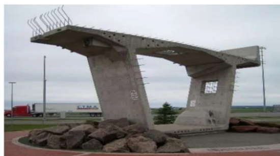
Fig 3. Display of a typical segment of the Confederation Bridge
